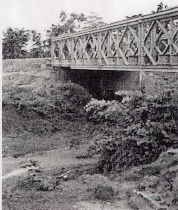
Bridge on the Kampong Speu-Oral District road, completed in April 2003
